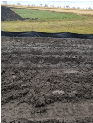
Access to 1071 ROW conditions Photo taken facing South
