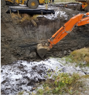
Excavator Ditching to 5.2 meters beneath the channel at Thornhill Coulee. Photo taken facing North East
