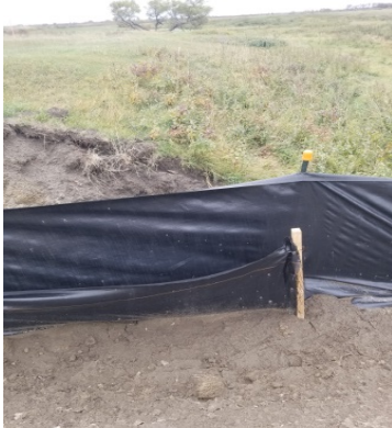
Silt Fencing installed at Thornhill Coulee Photo taken facing North
