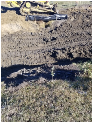
Backfill progress at Thornhill Coulee SSKP 1035.079 (MBR-WC3) Photo taken facing North
