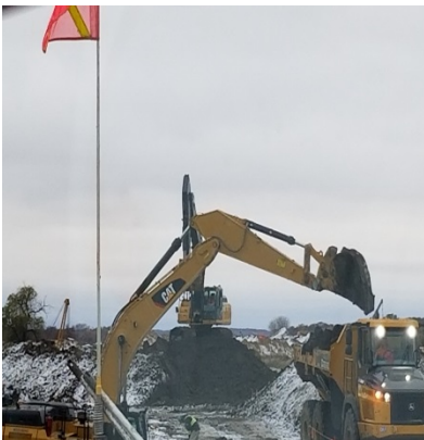
Excavator loading rock truck with soils from Thornhill Coulee to be kept separate Photo taken West
