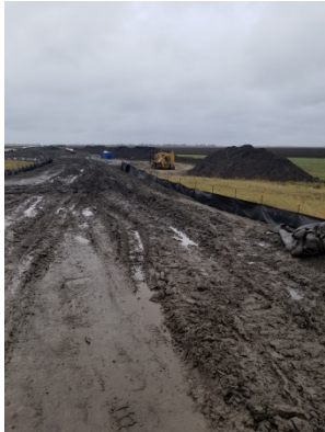
Access to 1071 bad conditions Photo taken facing East
