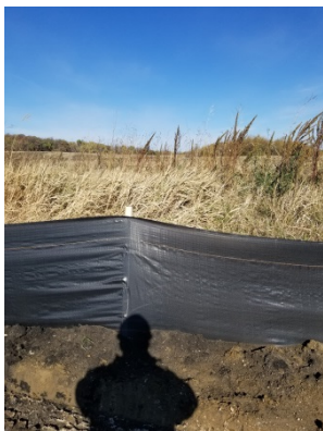
Erosion control (Silt fence) at SSKP 1014 (MB-189) Photo taken facing North
